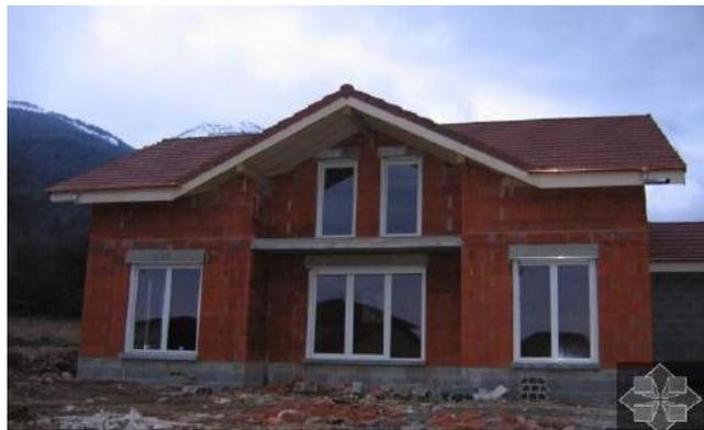
**Figure 3.** Masonry Load-bearing House.
