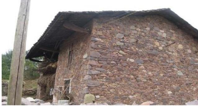
**Figure 4.** Stone Wall Load-Bearing House.
