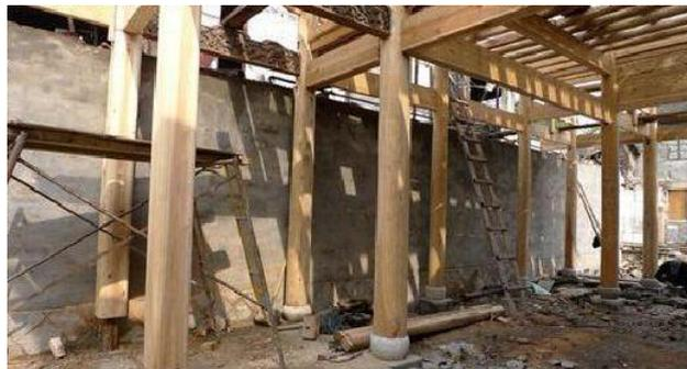
**Figure 1.** Wooden Framed Load-Bearing House.
