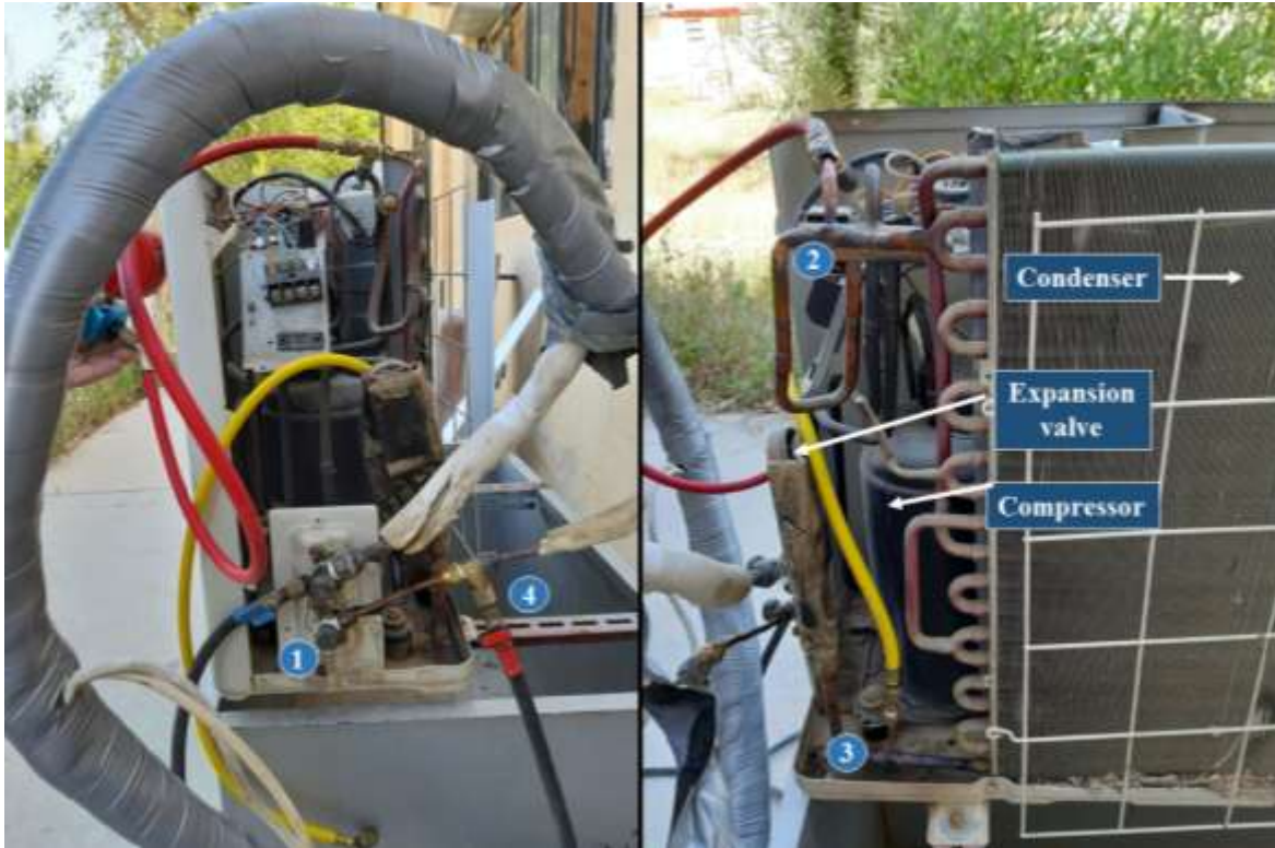
Figure 2: Gas gauge pressure location.
