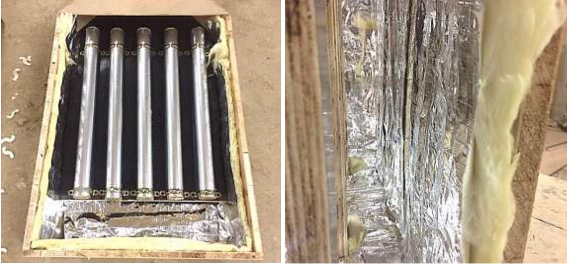
**Figure 2.** Insulate the sides and the bottom base with a thickness of 25 mm.
