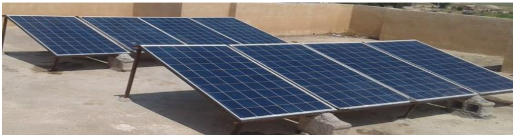
Figure 5. Shows the installation of the solar panel
