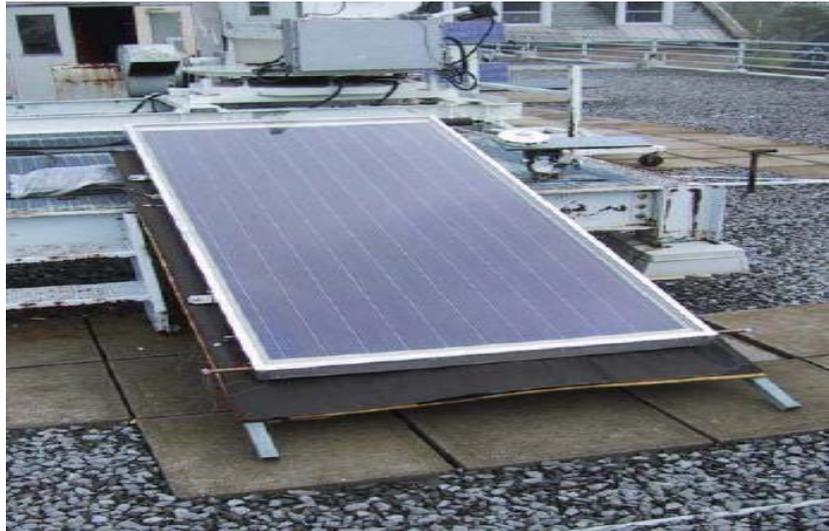
**Figure 2.** A planar solar collector
